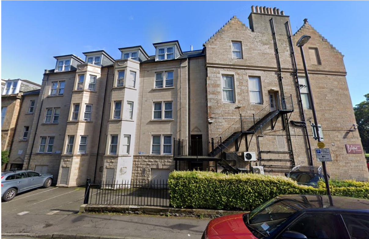
View opposite 86 Leamington Terrace
